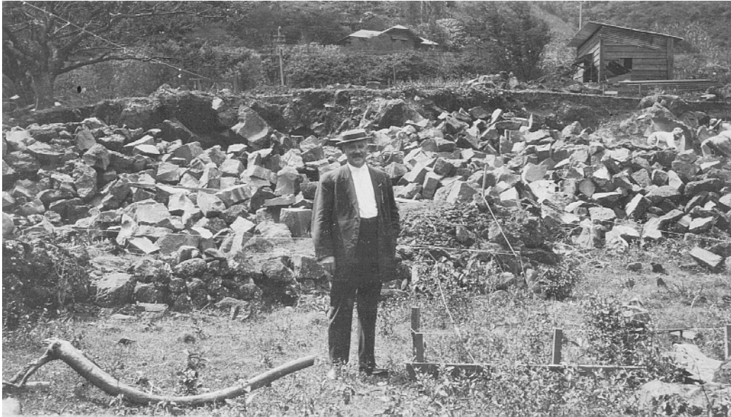
Photo 7. Blue stone quarried from the site, used for the house foundation and chimneys at either end of the house. (The name of the individual in the photograph is unknown.)
